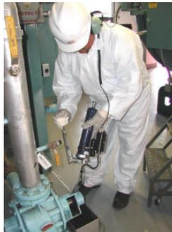
Traditionally, lubrication scheduling has been “time-based.” Equipment suppliers often recommend lubrication schedules based on hours of operation. In addition, they frequently provide instructions as to the amount of lubricant to be applied during these scheduled maintenance procedures.
