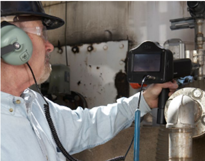
Figure 3 Inspector performing leak detection on critical facility equipment using the UE Systems Ultraprobe.
