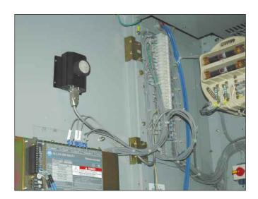
**UNIQUE FEATURES:** The UE-ECM 586 comes with an adjustable threshold level control. There are three outputs for your convenience: 4-20 mA, 0-10 VDC and Heterodyned (demodulated). The heterodyned output enables users to determine the cause of an elevated ultrasound level and record events through a typical audio recording device (MP3 recorder, computer, etc.).
