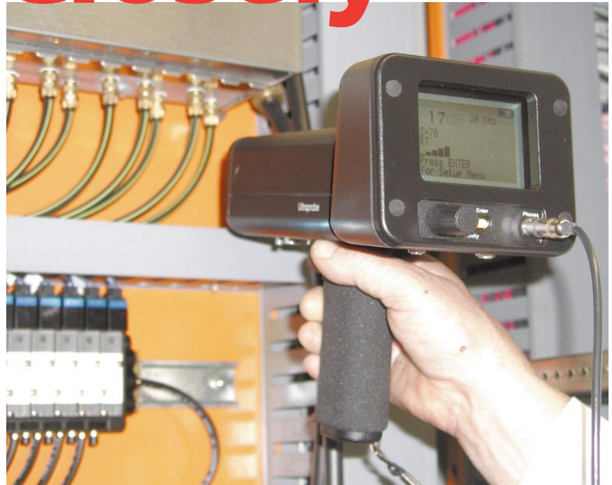
Ultrasonic technology can be used by maintainers to find pressure and vacuum leaks.
